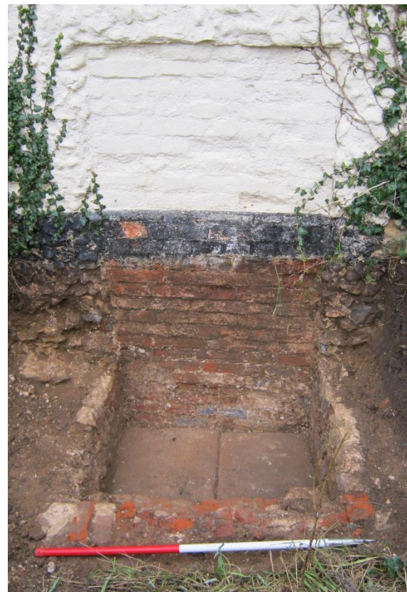
Plate 6: Sunken steps (17) to blocked doorway (looking north-west) [1m Scale]
